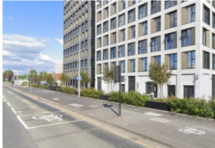
Fig.3.49 Today Broadway road has a shared path for cyclists and pedestrians.
